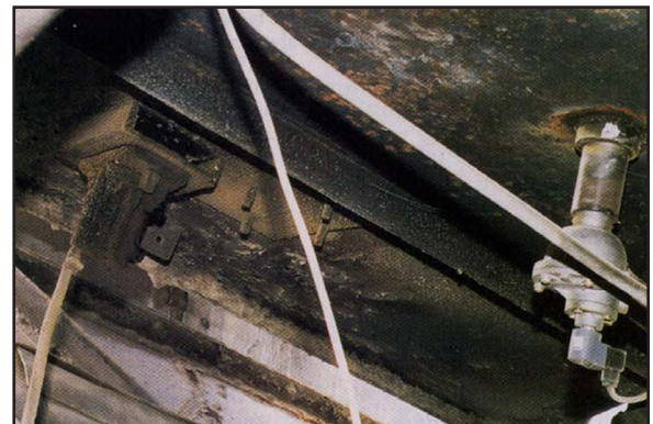
Past attempts to move fly ash with other equipment, such as the pneumatic vibrator shown on the left, proved ineffective. AirSweep unit is on the right.
