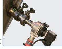
3/4" VA-06-TRI-TRI shown with solenoid valve.
